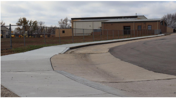
Figure 4: Beginning of the Sidewalk Project at the St. Elizabeth School 6
